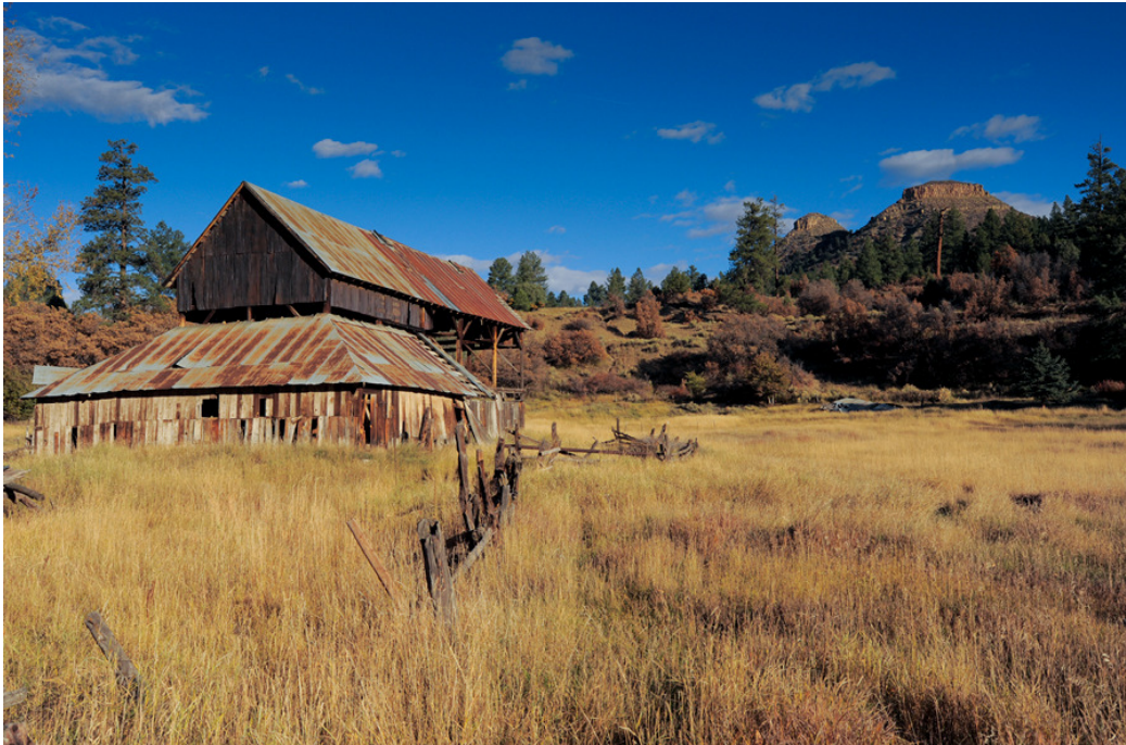
Exhibit 5. Historic Barn in the Twin Buttes Development.
