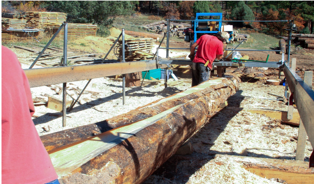
Exhibit 4. Construction Site in the Twin Buttes Development
