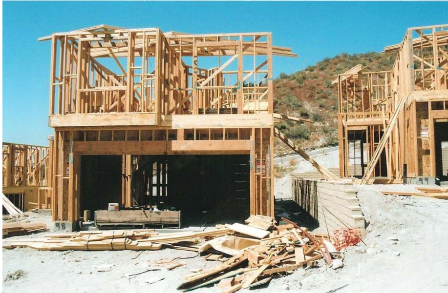
Above: Waste at a Wood Frame Job Site
